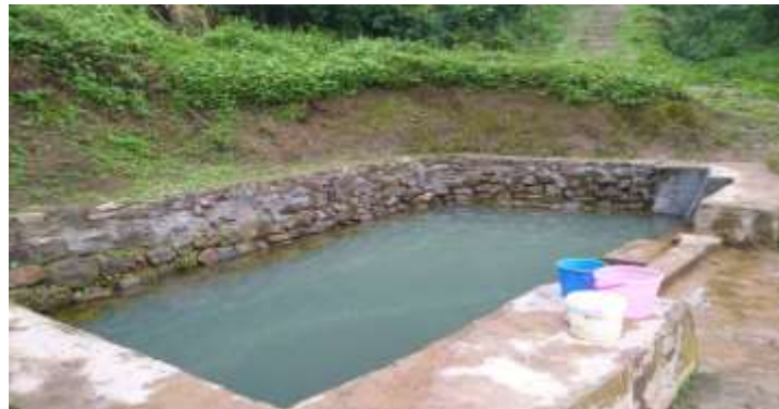
Figure 2: Spring water Harvesting Chekra, Awontang, Ukhrul town ( 21 \times 13 \times 4ft )
