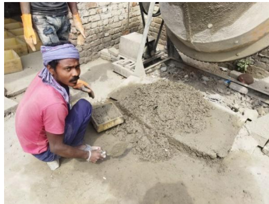
2. M-25 concrete mixing and fill up
