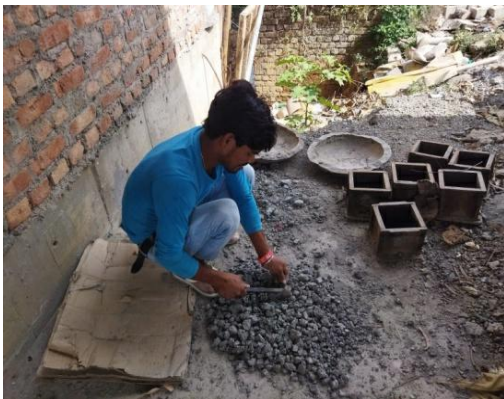
1. Wast concrete broken separately
