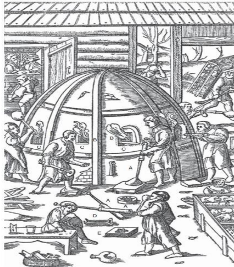
Fig4. Ancient furnace with windows for entry of raw materials and melting
