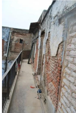
Figure 8 Corridor before restoration
