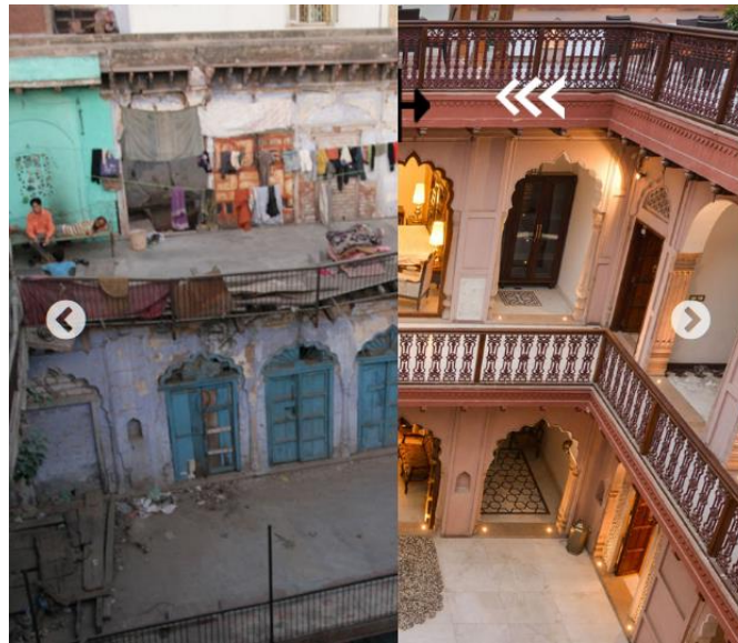
Figure 15 Courtyard before and after restoration
