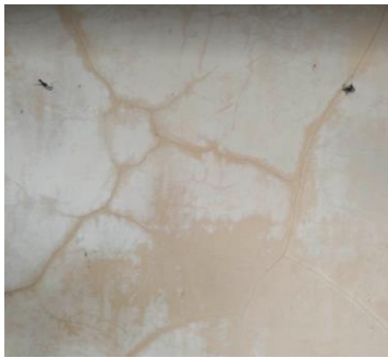
Hairline cracks
