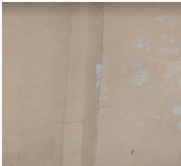
Hairline cracks
