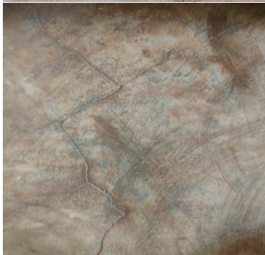
Hairline Cracks
