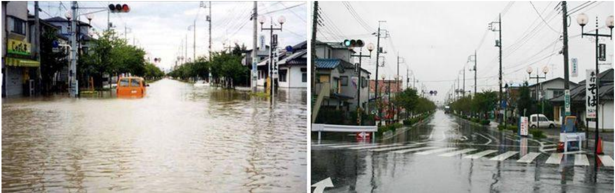
Fig 12: before and after the Discharge Tunnel was opened in 2004 right side and 2000 left side at saitama prefecture
