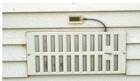
Fig. 9 OUTSIDE LIGHT SENSOR
