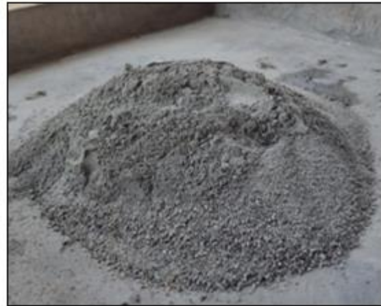
Fig.4.12 Mixing of cement and sand in a tray
