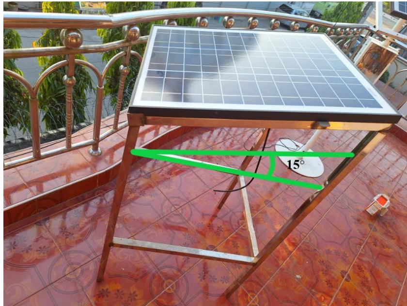
Fig (1) The optimal tilt angle in Myanmar is 15 degrees to the south
