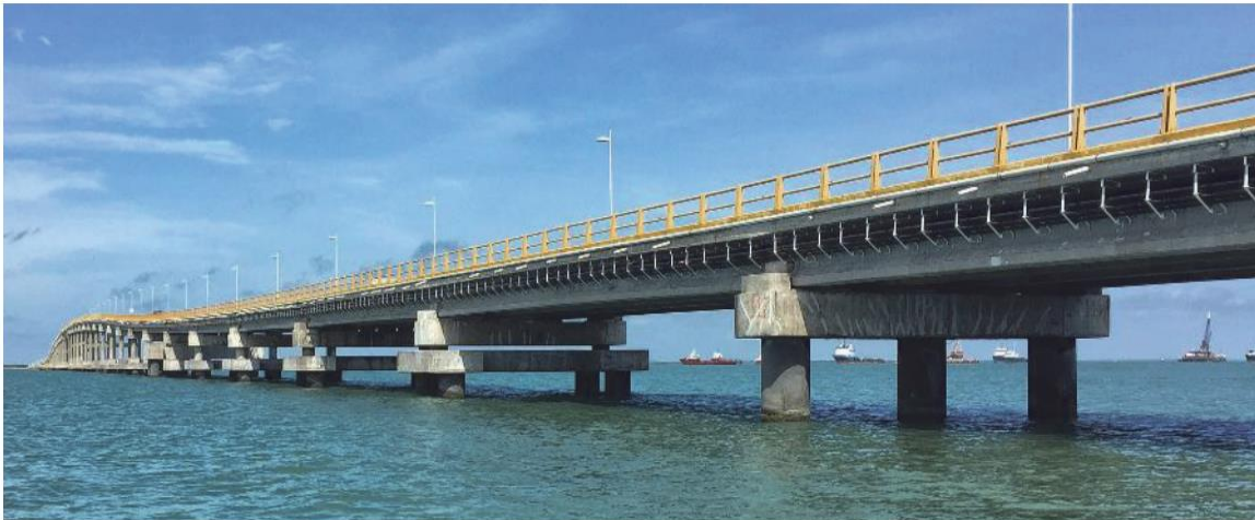
Figure 1.5: Bridge of pre-stressed concrete Girders el Zacatal, México [6].
