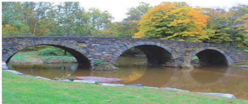
Figure 1.1 Bridge with stone arch design [3]
