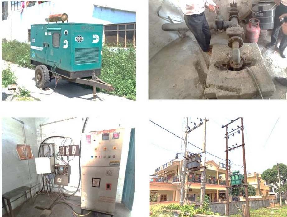
Figure 2: Existing pump house
