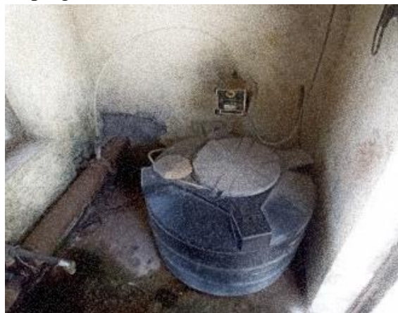
Figure 3: Chlorination unit
