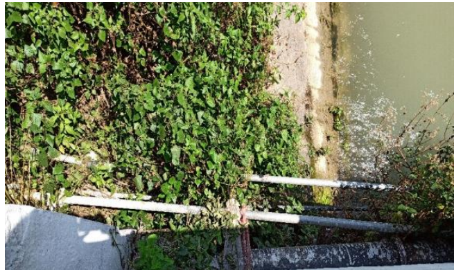
Figure 4: House service connections
