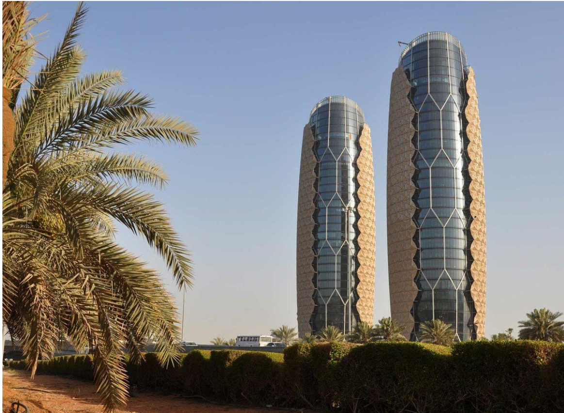
Figure 9. Al Bahr Towers
