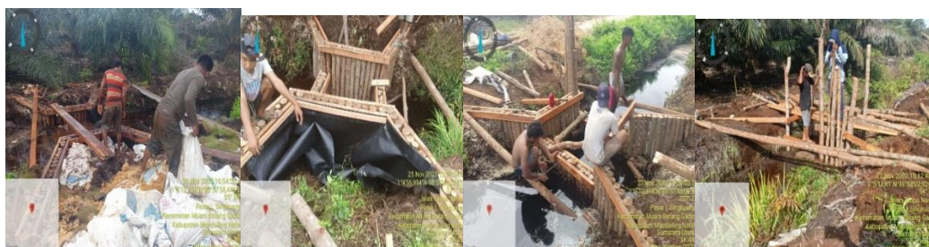
Figure 11. Construction work process of canal barriers
