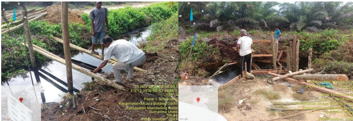
Figure 10. Land clearance and bow plank installation
