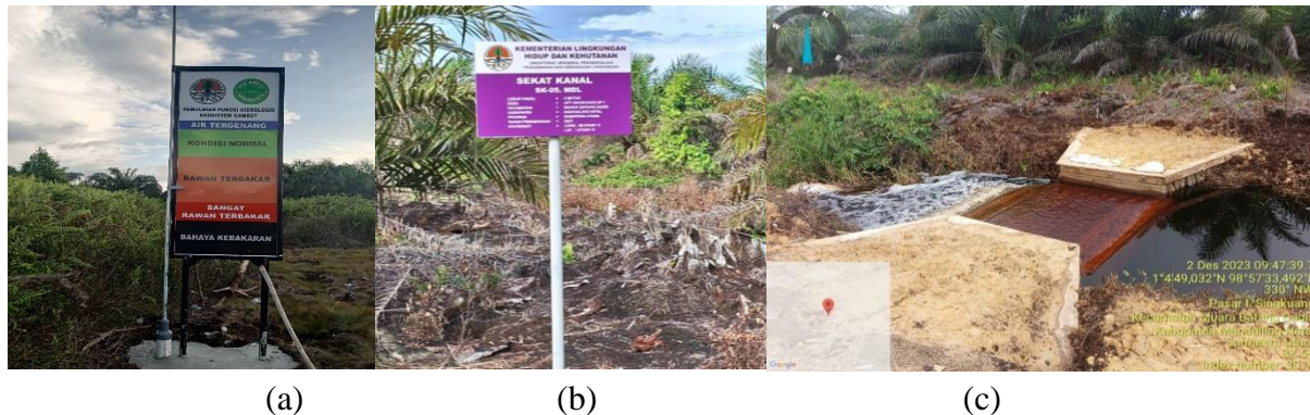
Figure 12. Final construction work of canal barriers.
