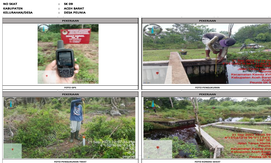
Figure 4b: Condition of canal blocks in West Aceh district
