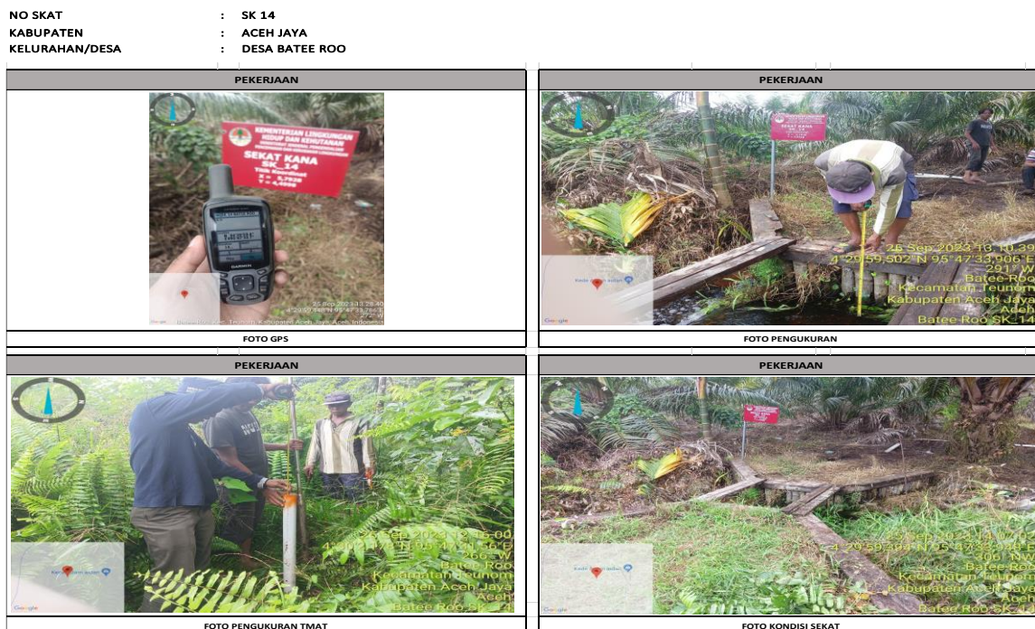
Figure 4a: Condition of canal blocks in Aceh Jaya district
