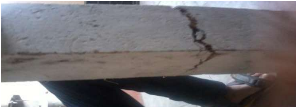
Figure 1.23: Cracking pattern coconut fibre reinforced concrete beam
