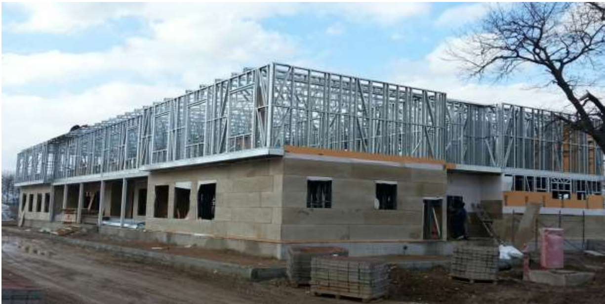
Fig 1.1 LGSS by CFS Structure (Istanbul) :
