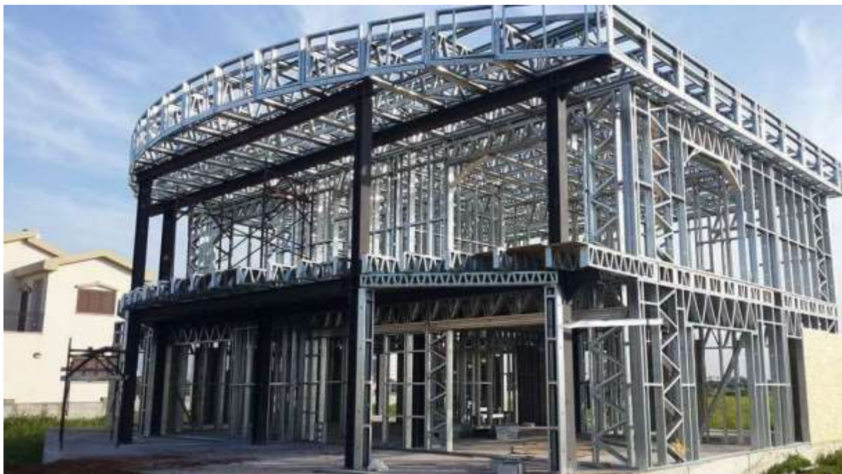
Fig 1.2 LGSS by CFS Structure (Istanbul):
