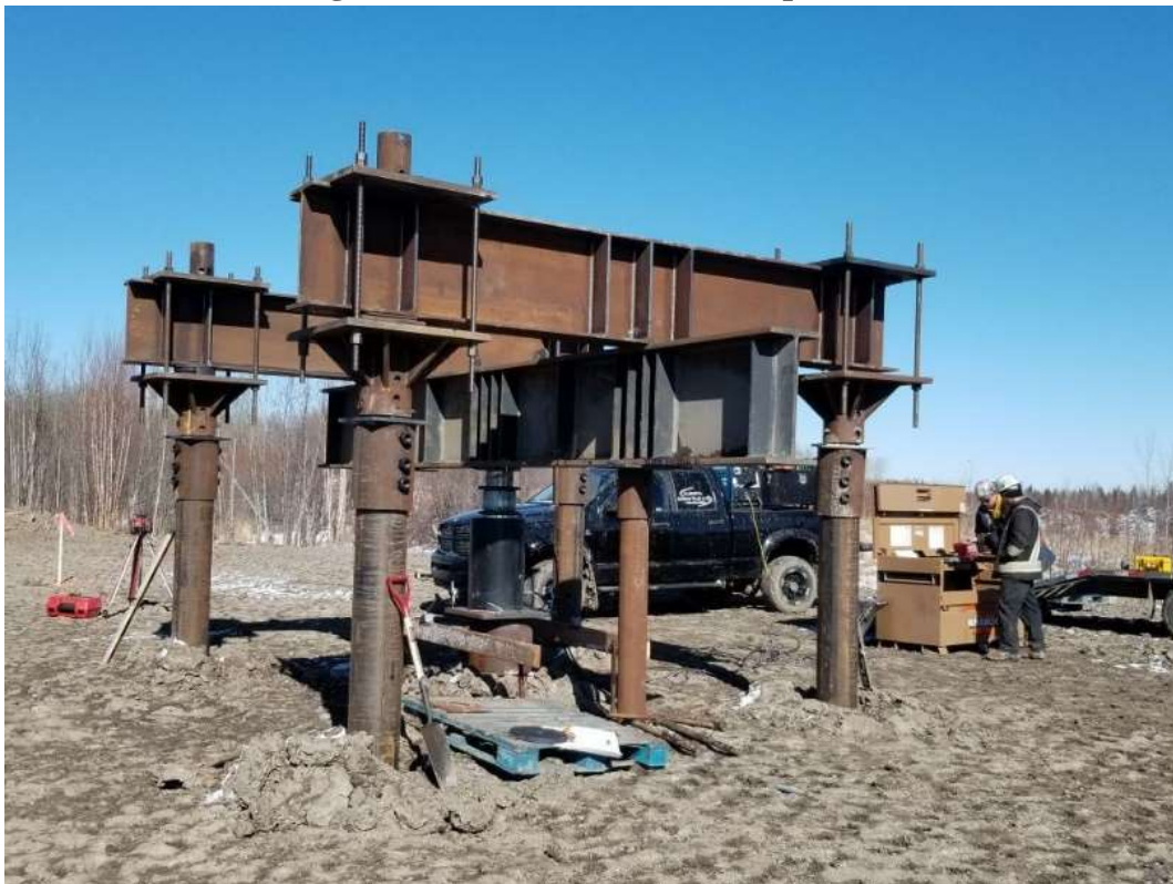
Figure 3: Actual Load Test Setup View
