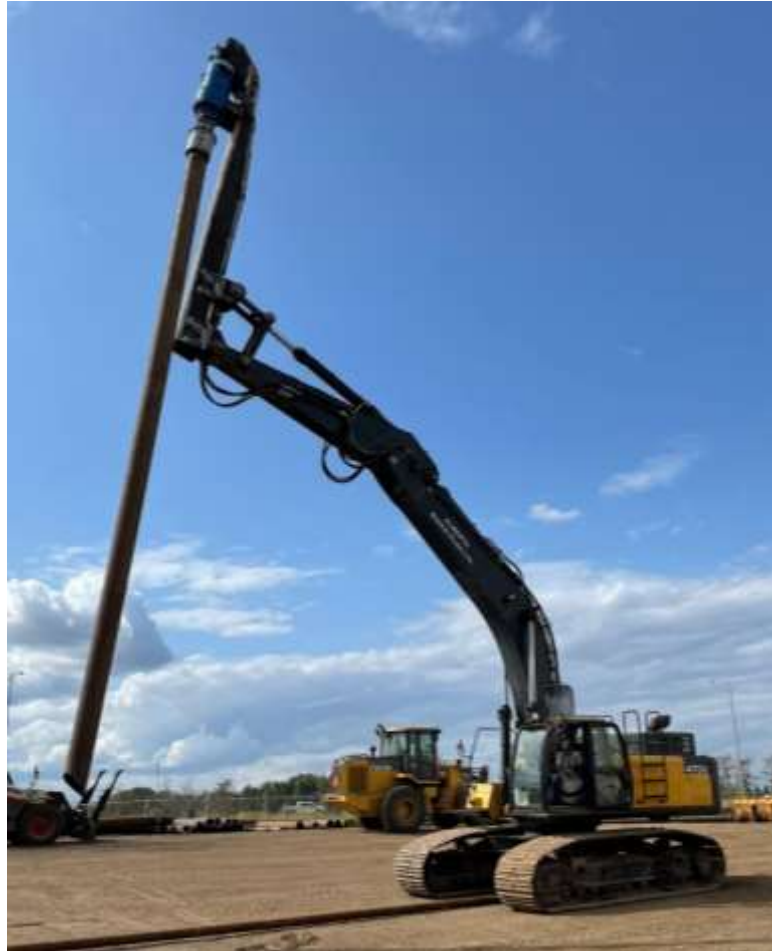
Figure 2: Typical helical pile installation unit
