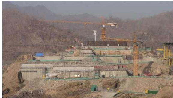
Figure 6 Site for SOU, Guj (During Construction)
