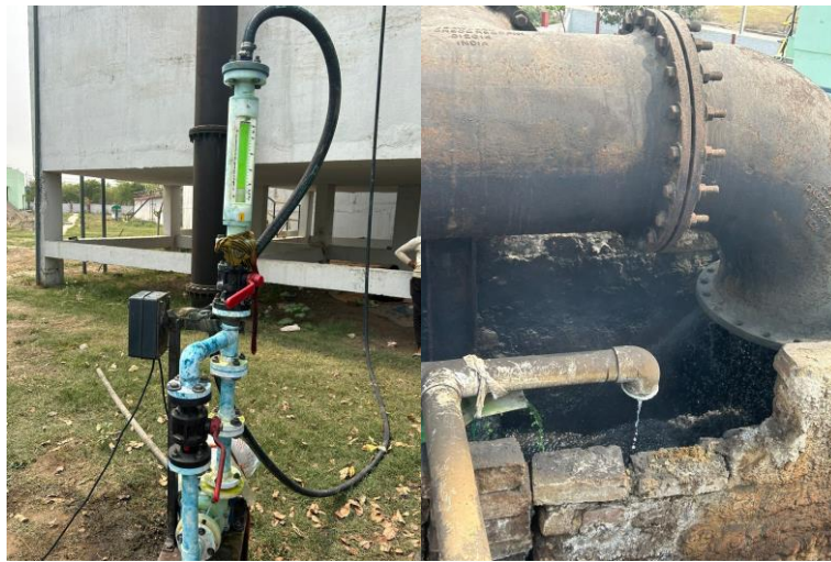
Left- Figure 1: PAC Pump brought in for a field trial
