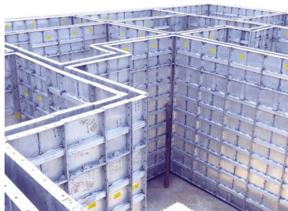
Picture 2: Formwork for Walls (Source-Walcoom)
