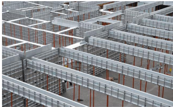
Picture 1: Formwork for beams (Source-Goldapple)
