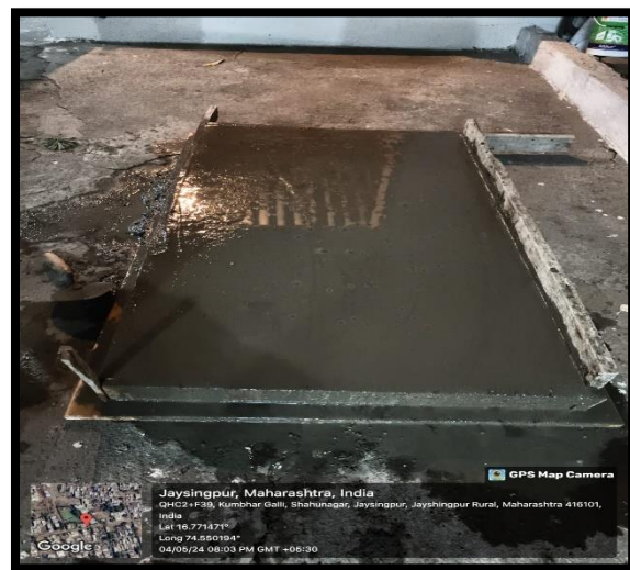
Concreting of slab- Use M20 grade of concrete
