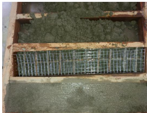
Figure 2. Picture showing placement of mortar mesh layers, and reinforcing steel bar.
