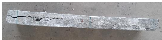
a. Bond anchorage failure
