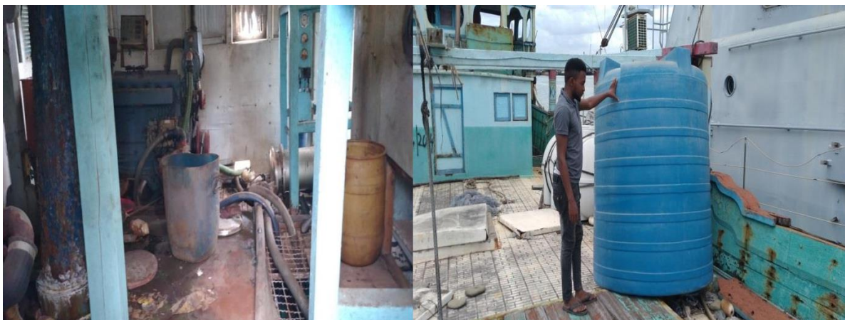
Figure 1.3 Empty tanks at police marine, Dar es Salaam
