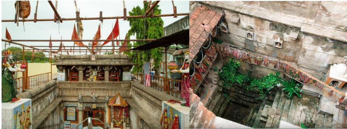
Figure 4 Some stepwells become deeply integrated into the life of their community, and it has become the embodiment of a living well. (Priyanka Sheth, 2020)
