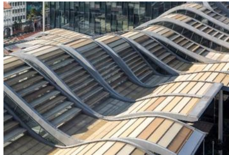
Figure 10: Louvers of the canopy reacting to sunlight (Partners, 2018)
