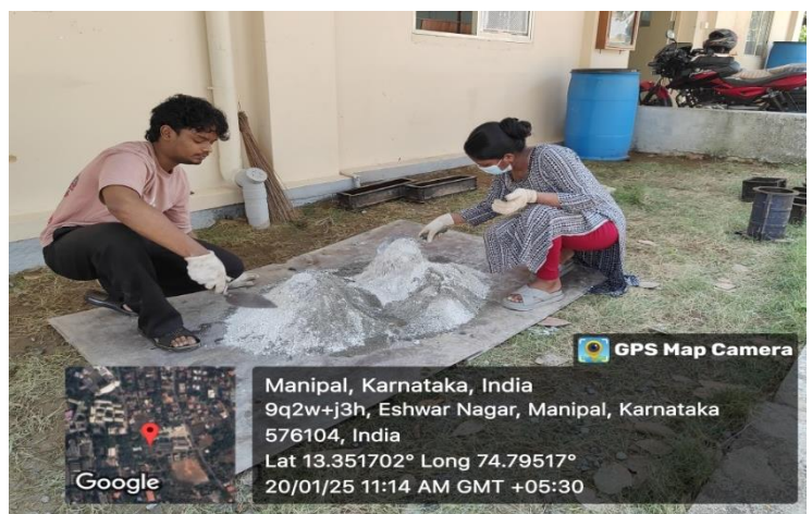
Mixing of Aggregates, Cement & GGBS
